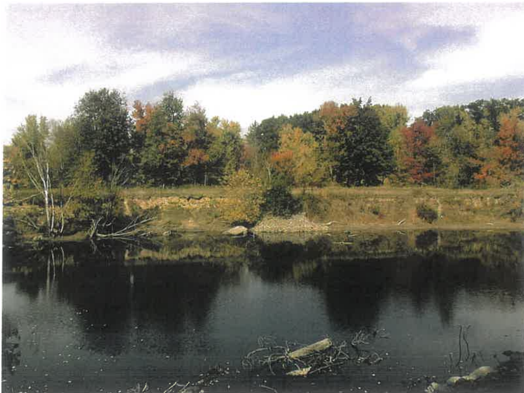
Photo 6 – Downstream left bank erosion
